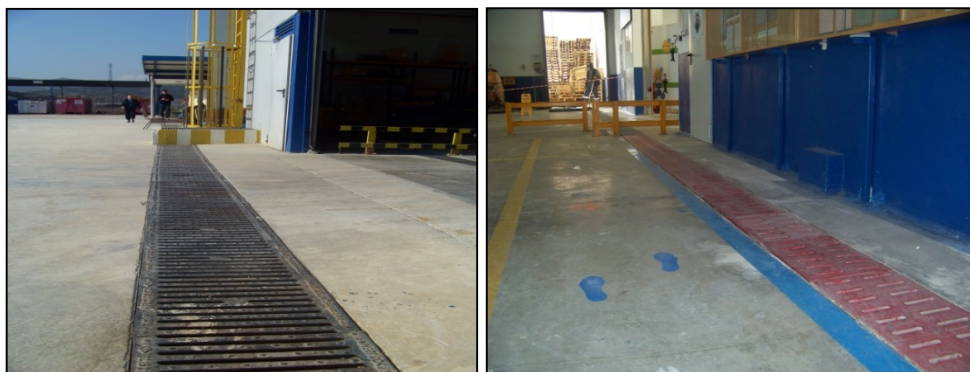
Figure 7a and 7b. The water tunnels that separate the water used and the rainwater in the production area
