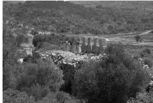
Fig. 6. Parapet and merlons that retain traces of insitu Seljuk paintwork
