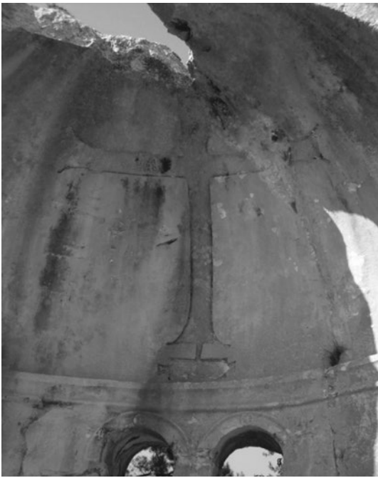
Fig. 11: Detail of the rock-cut apse of the Alacahisar Church.
