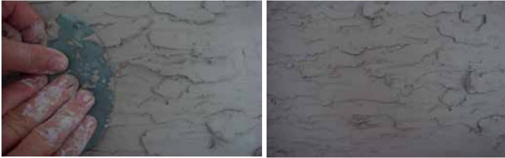
Figure 3: Form retouched by grinding
