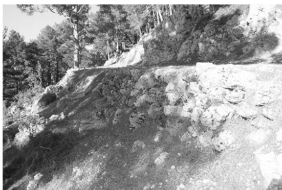
Fig. 24) Retaining walls of the road at Duman Pass.
