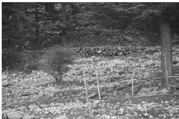
Fig. 22) Retaining walls of the road between Duman Spring and Duman Pass.
