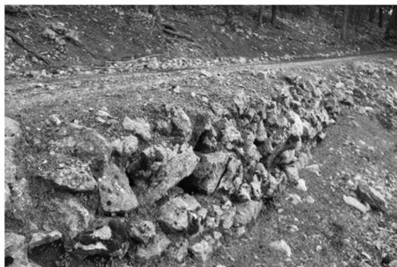
Fig. 23) Retaining walls of the road between Duman Spring and Duman Pass.
