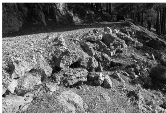
Fig. 25) Retaining walls of the road at Duman Pass.
