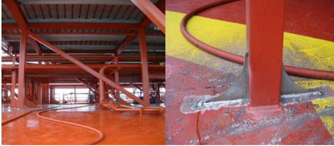
Figure 19. The applied repair / modification details on helicopter supporting structure [7].
