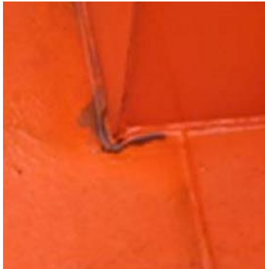
Figure 9. Crack in way of deckhouse corner [1].
