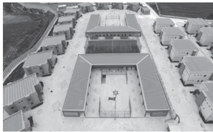
Figure 15: Final condition of the project
