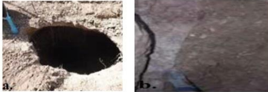
Figure 1a. View of the Sinkhole found in the South of Esentepe
