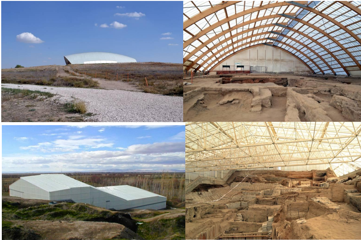
Figure 11 a-b: The shelter of 4040 area (North Area) (from authors archive)
