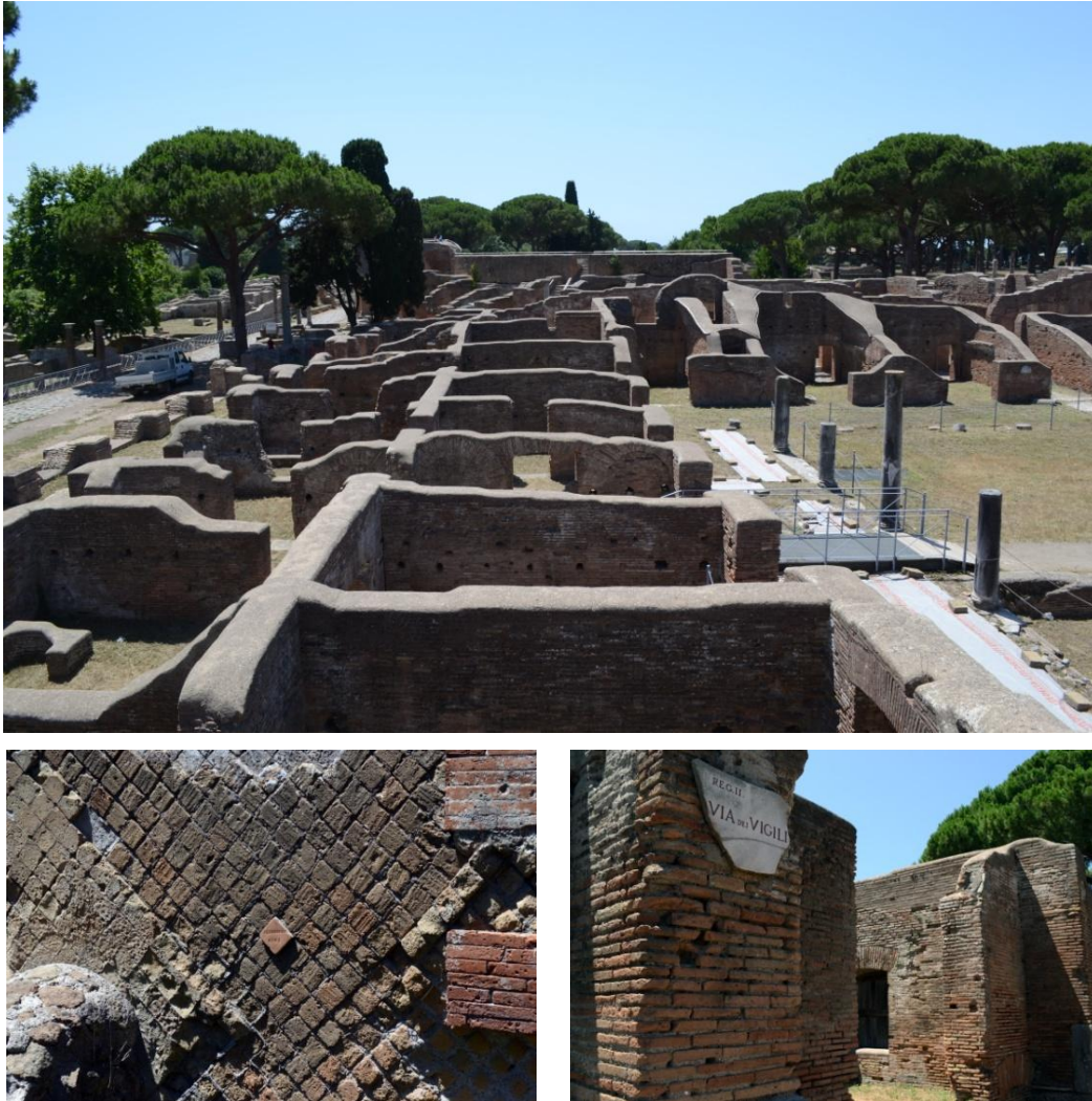
Figure 18 a-b-c: Intervention techniques in Ostia Antica, 2016 Source: Authors Archive
