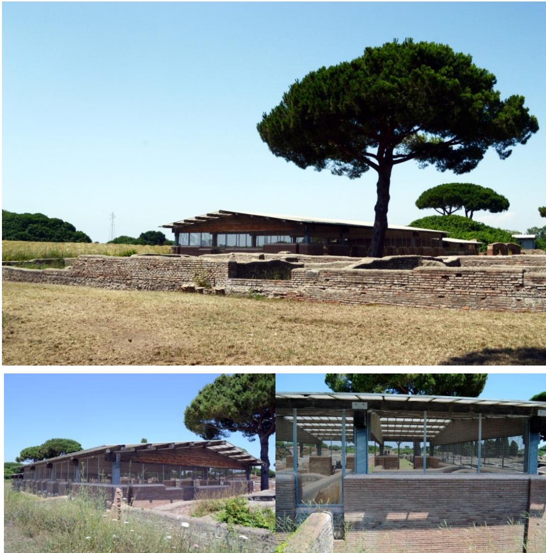
Figure 19 Protective Shelter Source: Authors Archive
