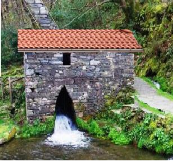
Figure 2. A view of micro-water structures in the Eastern Black Sea region (Watermill).
