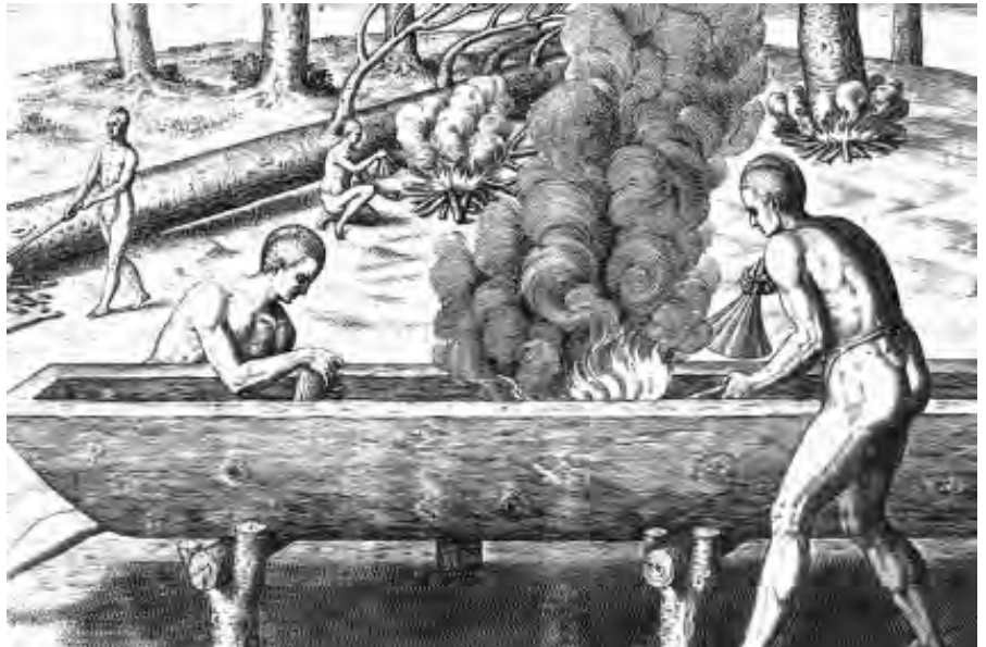
Figure 10 A late 16th century drawing of hollowing a dugout by fire method (after McGrail 2001: 423 fig. 11.25).
