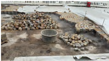
Figure 7 Laying the pavement, Trier ©MJ Duran Kremer.
