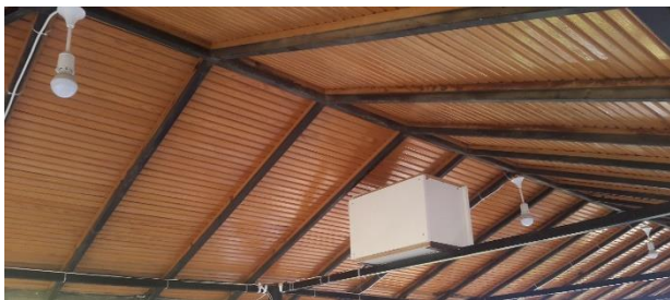
Figure 3. Charging and Wireless Data Transfer Station
