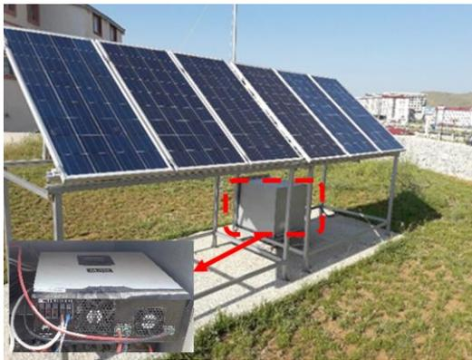
Fig. 2. PV panel and inverter
