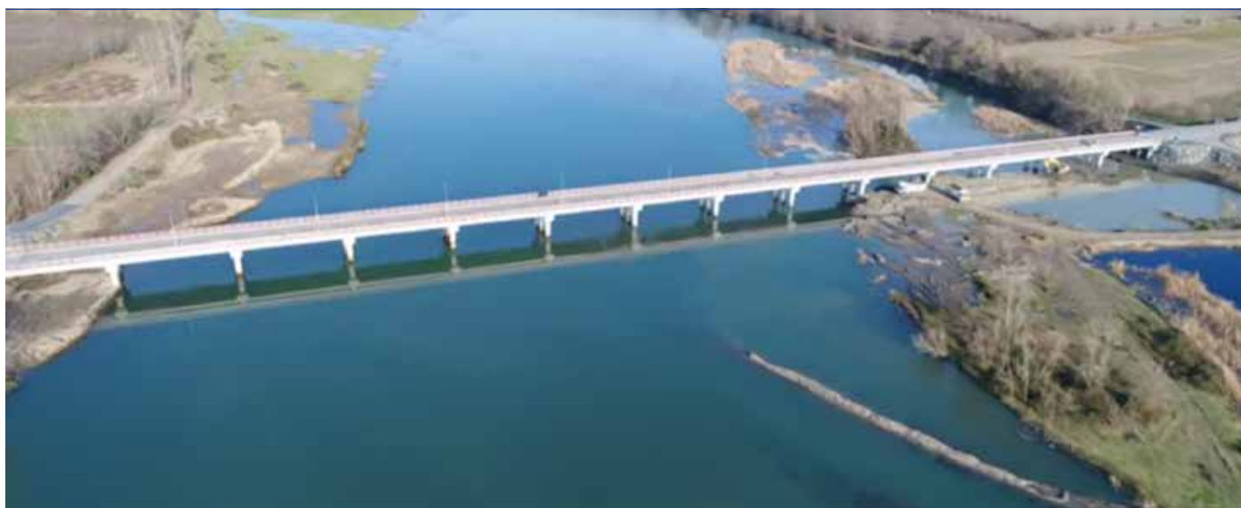
Figure 6. A view of Hürriyet-Kumtepe Bridge on Yeşilırmak (Photo: https://www.youtube.com/watch?v=LB2XsnuGjZU )
