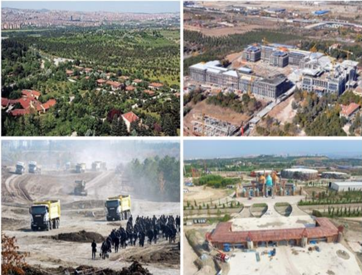
Figure 7. AFF's previous green spaces and the status of after it is occupied for constructions (Anonymous, 2017d).
