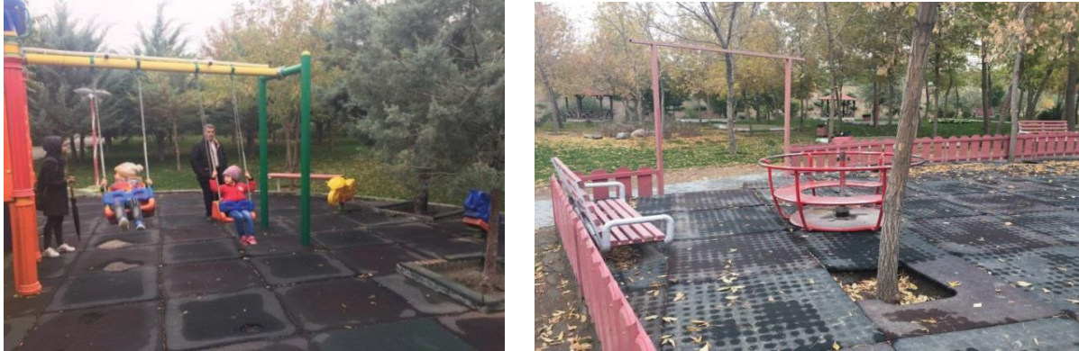
Figure 18. Stripped playground covering in the Autism Park stripped (left) and formation of level difference in the First playground (right) (Aysan Danesharasteh's personal archive)
