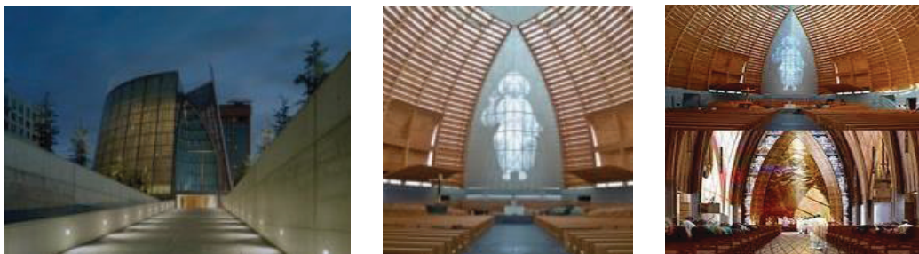
Figure 5. Cathedral of Christ the Light – the cathedral made of wood and glass in Auckland California [URL 6]
