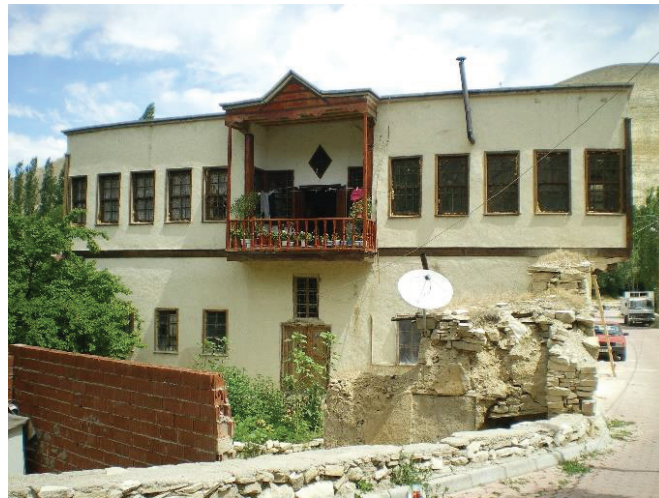
Figure 7. In Gürün, the building constructed in an incompatible manner with the architectural texture in the garden area of Hüsrev bey Residence (2014)
