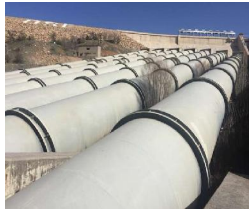
Figure 1. Penstock pipes
