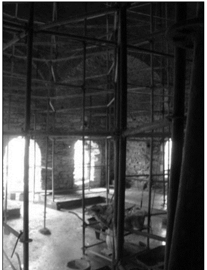
Fig. 8 Repairing of jointing
