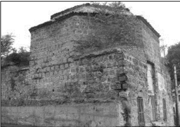
Fig. 2 West and south façades
