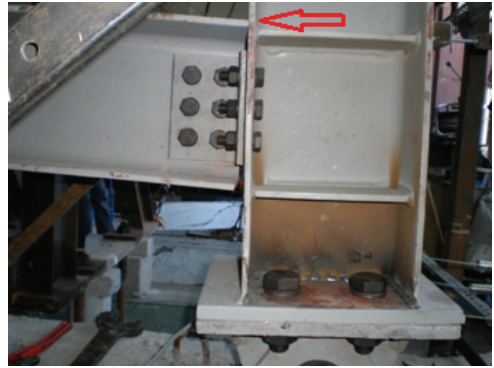
Figure 18 - Beam flange in the connection coming into contact with the column
