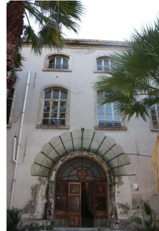
Fig.7: Entrance Façade of the Main Factory Building-2015
