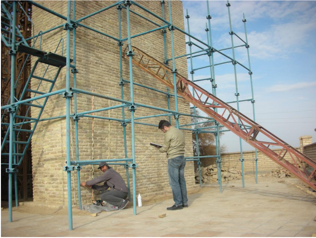
Figure 2. A representative application on tower walls.
