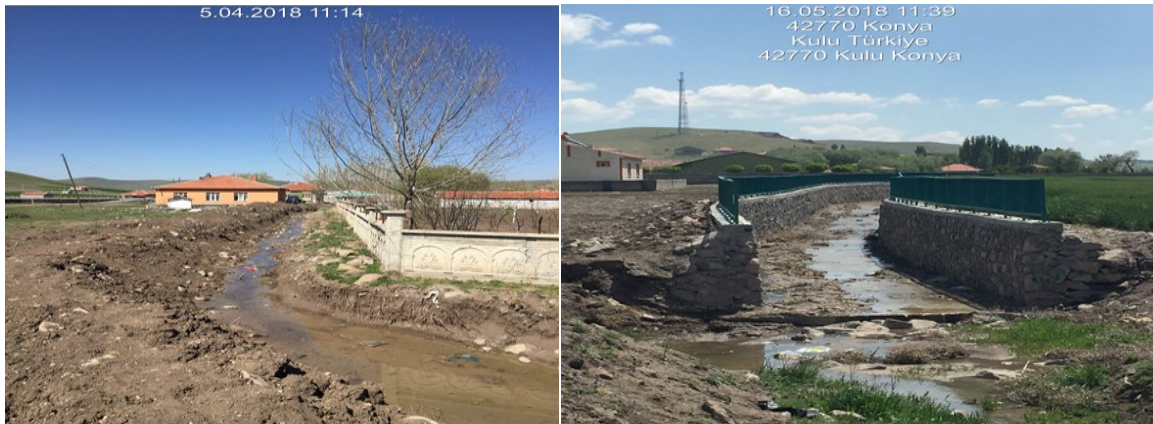
Figure 5. Flood protection plain of Kulu
