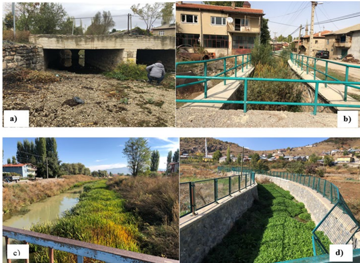
Figure 9. Narrowing of the cross-section by planting in a) Akcalar region, b) Harmanpinari region, c) Esence region, d) Bagbasi region
