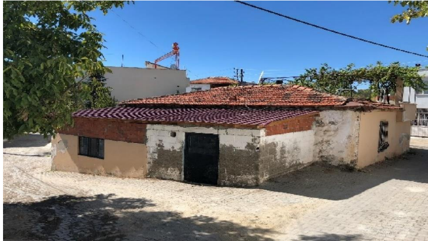
Photo 6. An example of traditional house in Kavlaklar
