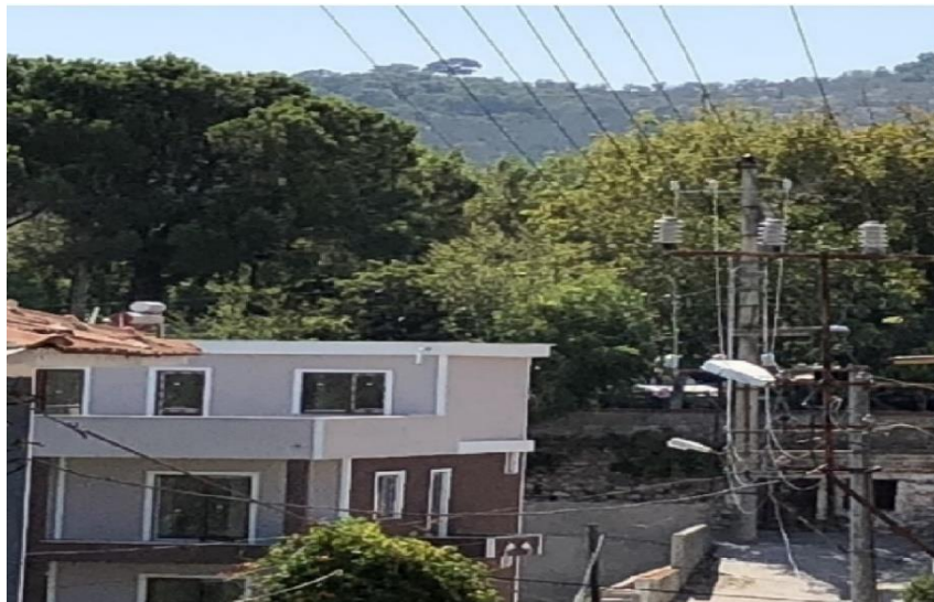
Photo 5. A photo of urban reconstruction in Kızılköçü
