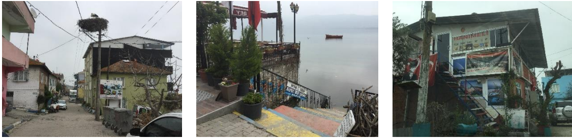
Figure 9. Bad condition of traditional dwellings due to improper use, such as being fish restaurant and café (source: Authors 2017)
