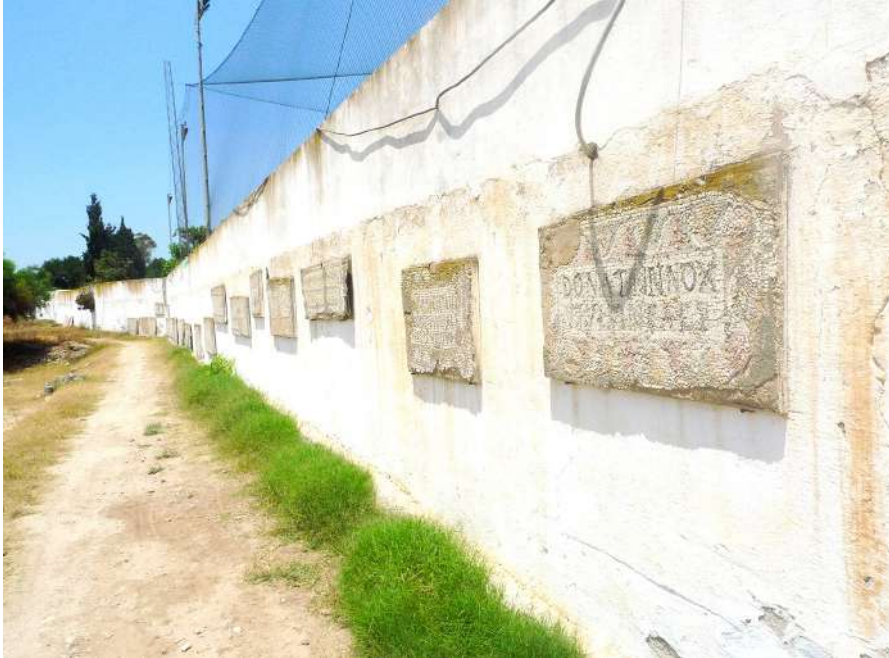
Figure 21 Puppit (Souk el-Abiod), clôture du site (photo J.Hajji).
