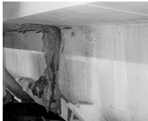
Figure 2. Steel leakage through tundish wall due to carryover slag erosion
