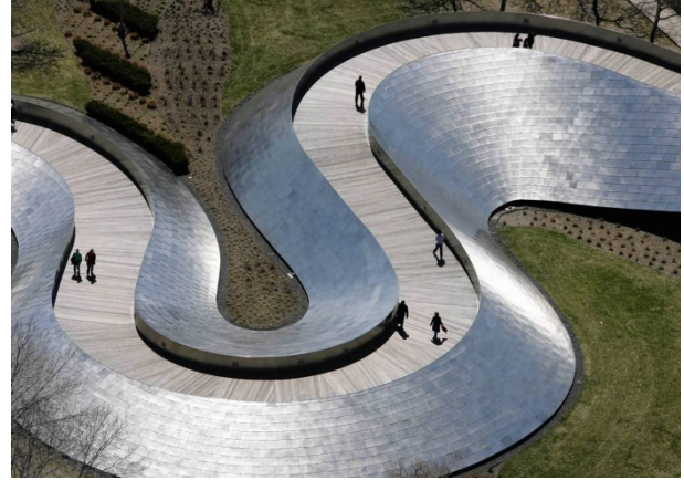
Şekil 25. Millennium Park BP Pedestrian Bridge, Chicago, ABD
