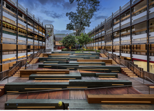
Şekil 31. Enabling Village, Redhill, Singapur
