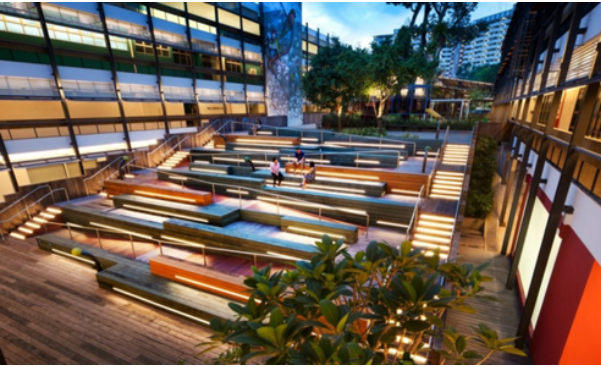
Şekil 32. Enabling Village, Redhill, Singapur
