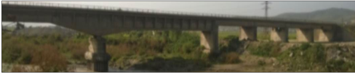
Figure 8. Photo of the bridge.
