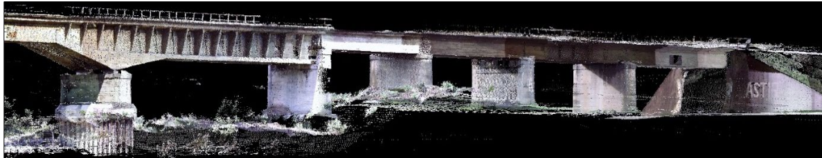
Figure 9. Isometric view of the bridge obtained from the cloud of colored points with terrestrial laser scanner image.
