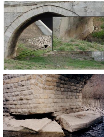
Figure 9. Trabzon, Macka road Mataraci Bridge
