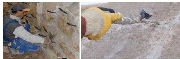
Figure 12. Injection application
