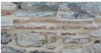
Figure 15. Reconstruction of the demolished part with mortar
