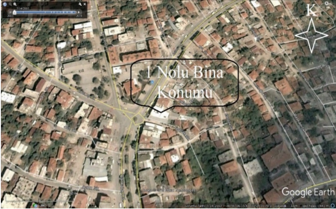
Şekil 4. 1999 Adapazarı Depreminde Devrilen 1 Nolu Binanın Konumu, [2] (Location of Building #1 Which was Overturned in 1999 Adapazarı Earthquake)
