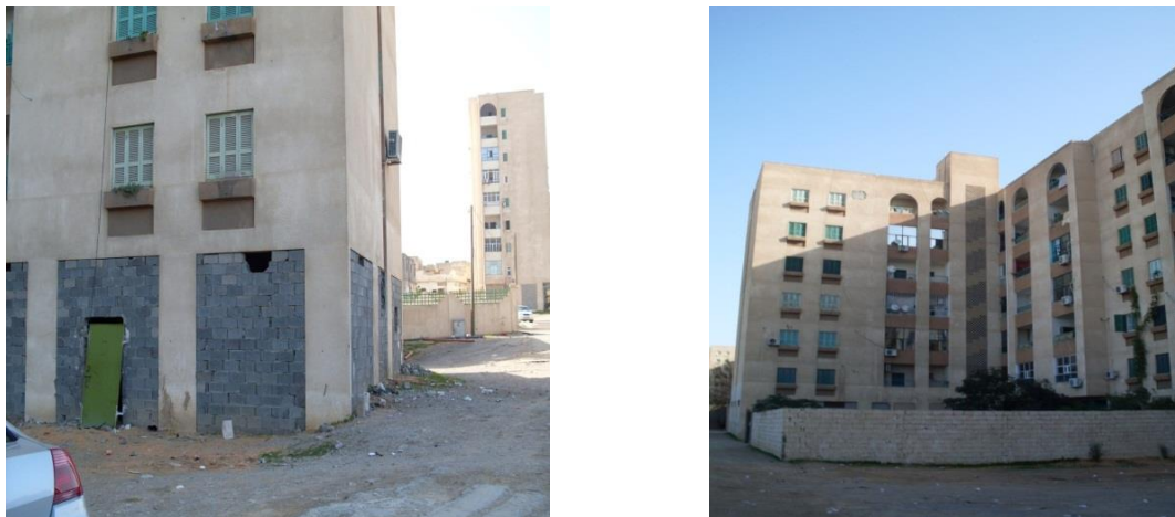
Figure 7. A number of changes on the ground floor (left) and neglect of the site environment of residential buildings by users (right) (Source: O. A. Alameen archive)
