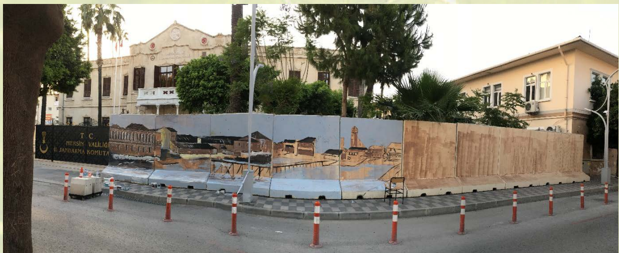
Photo 12: Mersin Urayart 2019 “Gendarmerie building, security wall” 2019
