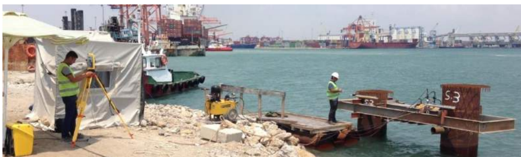
Figure 7. Lateral Load Test Set-up
