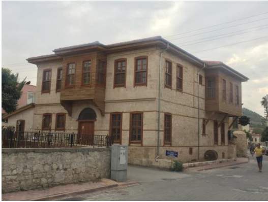
Photo 5: Restored registered building
