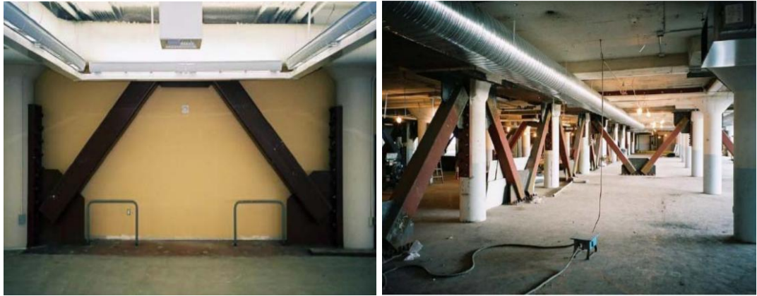
Figure 2. Steel brace applications (Yon and Sayin, 2011)
