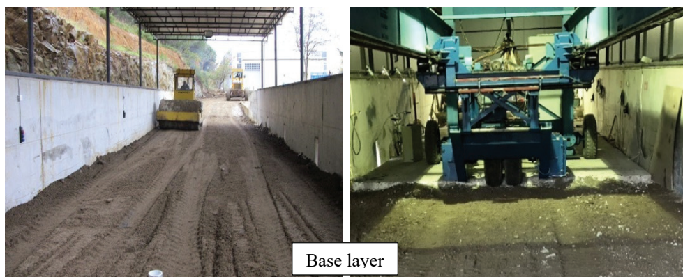
Figure 5 - The base layer beneath the concrete pavement
