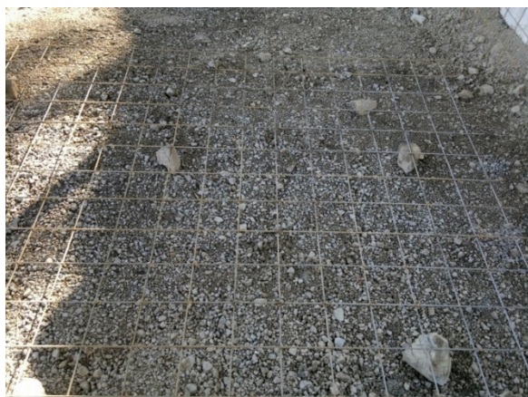
Figure 4 - Mesh reinforcement was positioned 60 mm above the base layer
