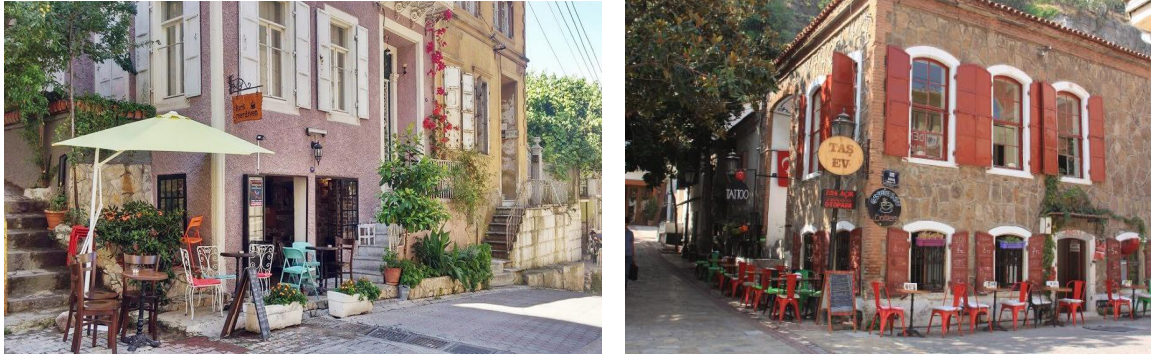
Figure 6. Some of the public spaces in the settlement
