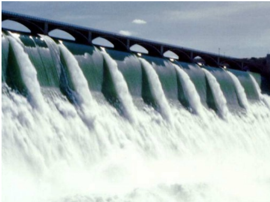
Figure 2. Hydroelectric Power Plant (HEPP)
