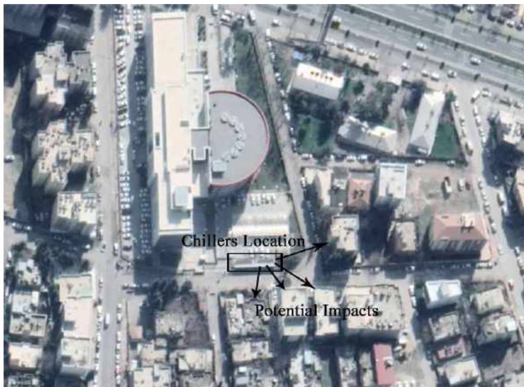
Figure 3. Location of the chillers with respect to neighboring family houses.
