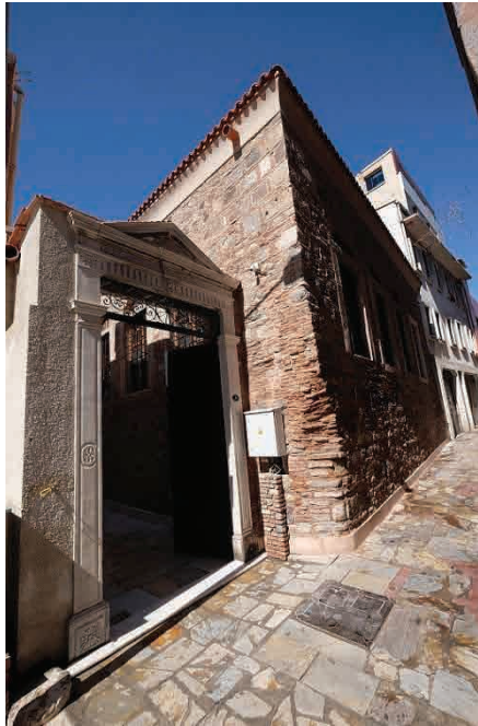
F. 12. Post-restoration, southern façade and courtyard entrance (Mehmet Yasa, 2018)
