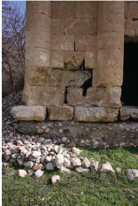
F. 17. The exposed foundation concrete (Kemal Kutgün Eyüpgiiller, 2018)
