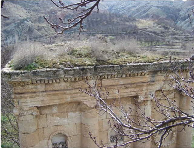
F. 7. Northern view of the roof (Kemal Kutgün Eyüpgiller, 2018)
