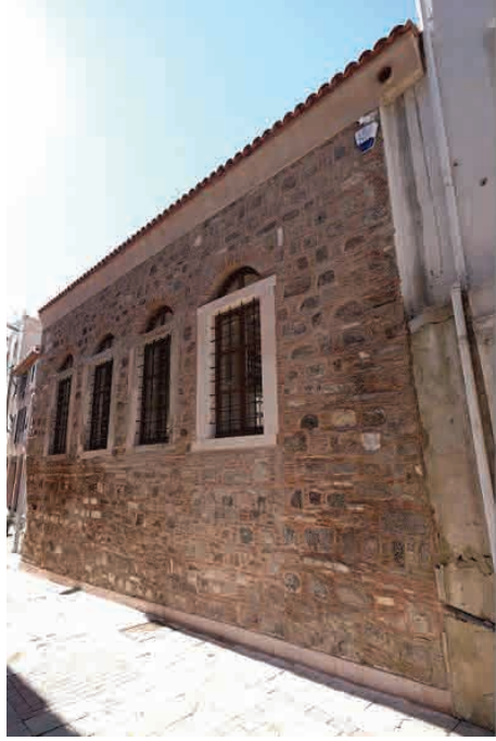
F. 13. Post-restoration, southern façade (Mehmet Yasa, 2018)
