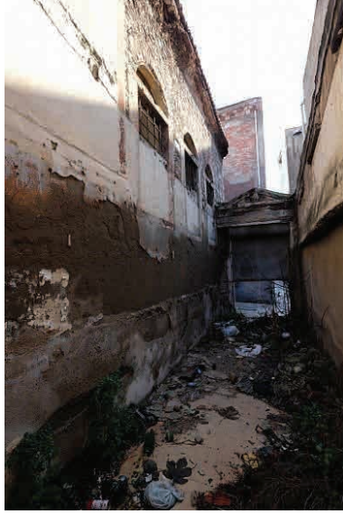
F. 4. Pre-restoration, courtyard and western façade (Mehmet Yasa, 2017)
