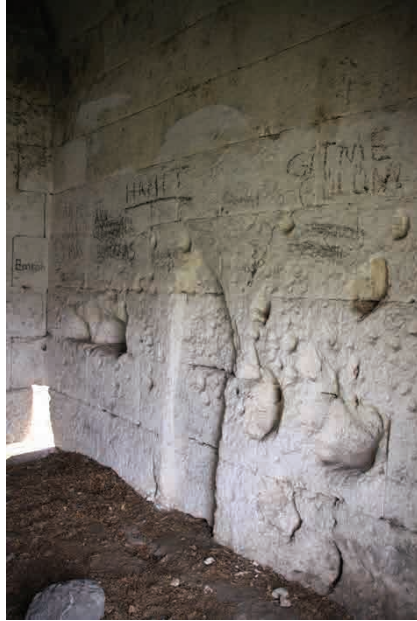
F. 13. The interior surface of the south wall, the mihrab-like niche and the original floor (Kemal Kutgün Eyüpgiller, 2018)
