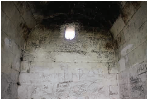
F. 19. The interior surface of the east wall (Kemal Kutgün Eyüpgiller, 2018)
