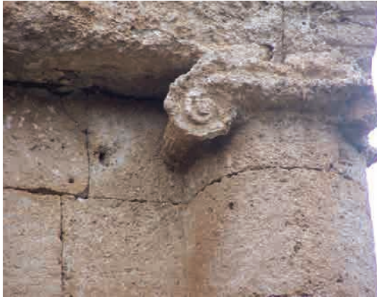
F. 18. Surface loss on the column capitals (Kemal Kutgün Eyüpgiller, 2018)
