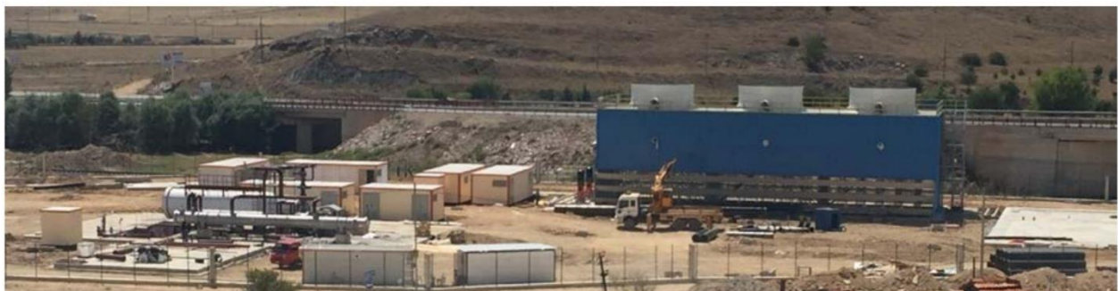
Figure 1. A general overview of Afyon Geothermal Power Plant (AFJES) (Sahin, 2016).
