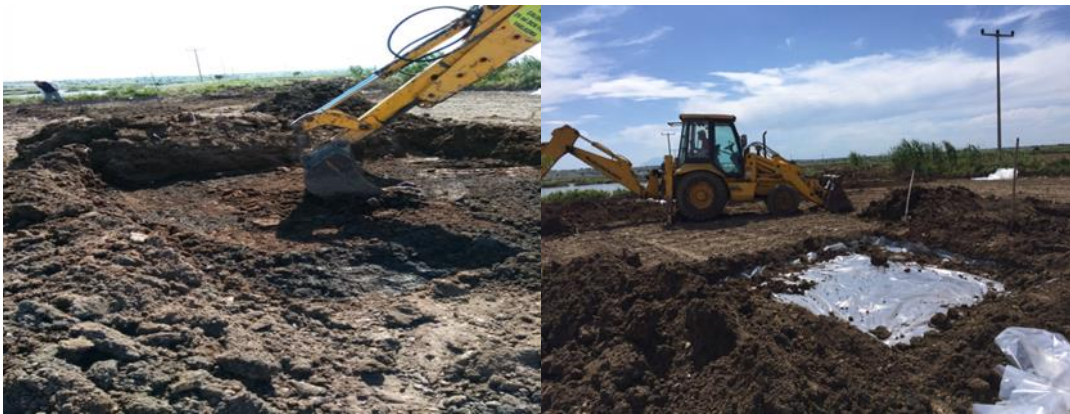
Figure 2. The excavation for water retention barriers
