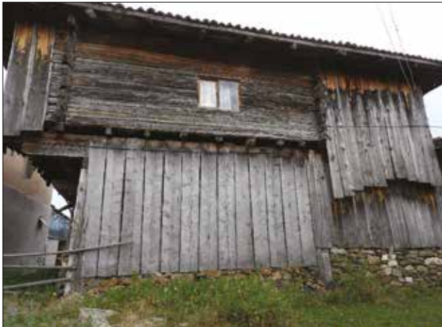
Fotoğraf 44. Darabalı zemin kat, Terzi Ahmet Köyü, 2018 / Ground floor with darabas, Terzi Ahmet Village, 2018.
