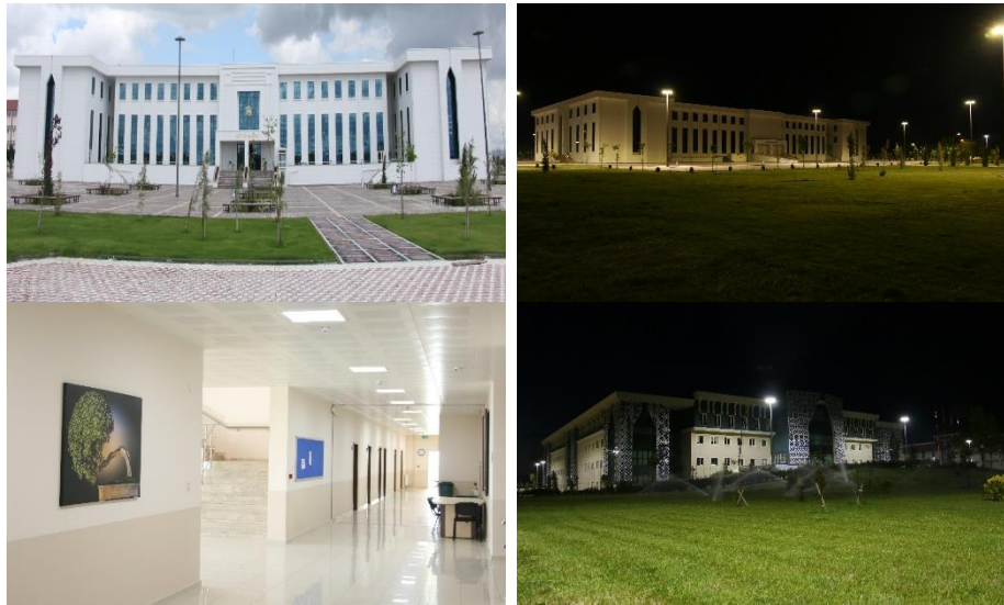
Figure 6. ASU library (green building example) and lighting systems
