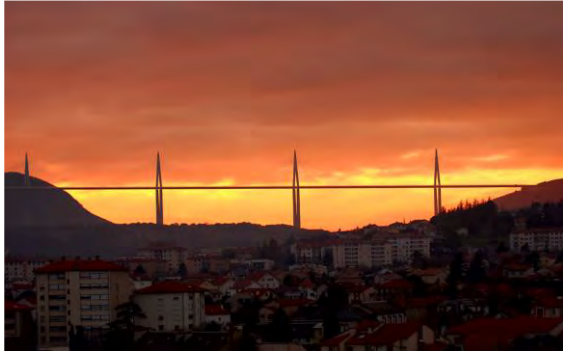
Figure.8. Millau Viaduct, France, 1993-2004 ) ( www.fosterandpartners.com )
