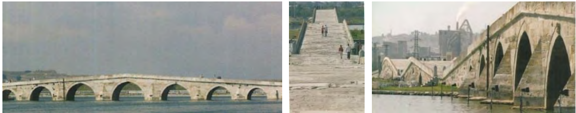
Figure.4. Views from Büyükçekmece bridge, (Necipoğlu G, 2005)
