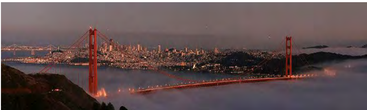
Figure.6. San Francisco with two bridges (Western section of the Bay Bridge in the left background),Coit Tower (in background to the left of North tower),and Fort Mason (on the San Francisco waterfront in the background behind the North tower) from Marin. (source: http://goldengate.org/exhibits )
