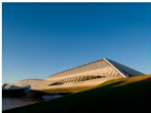
Figure.12. Exteriors views of the bridge-pavillon, ( http://www.zaha-hadid.com/design/zaragoza-bridge-pavillon/ )
