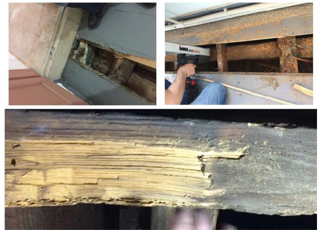
Figure 3. Evaluation of the beams by Resistograph.
