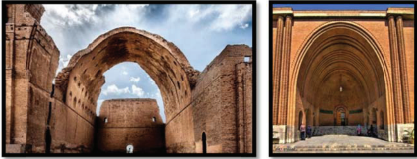
Figure 5: Left to right: the historic Sassanian Ctesiphon Vault, the entrance of the National Museum of Iran 3233
