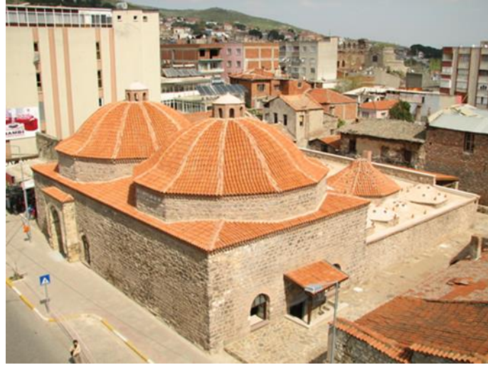
Figure 1. Example of a Turkish bath with a square plan and dome (Bergama Hacı Hekim Bathhouse) (Anonymous, 2016)
