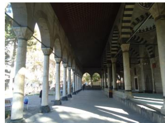
Figure 58. Kurşunlu Mosque Northern Façade (Hasözhan, 2016)
